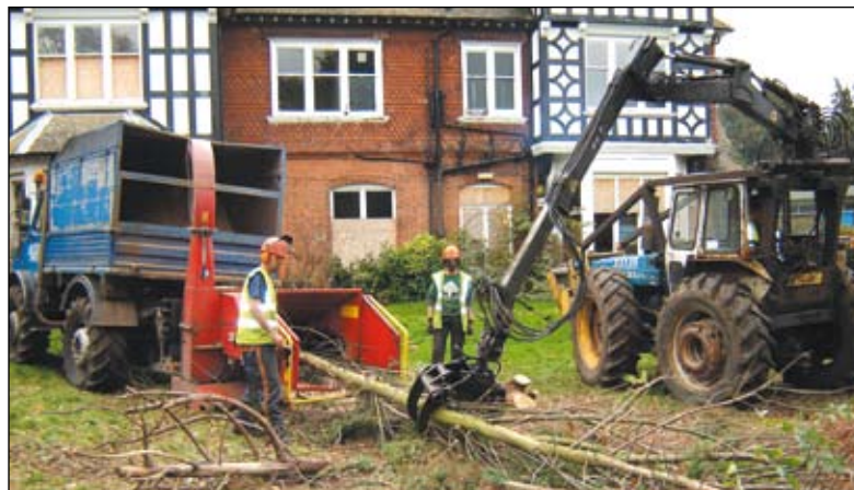
The County 1164 feeding the TP 250 on a site clearance at Croydon.
