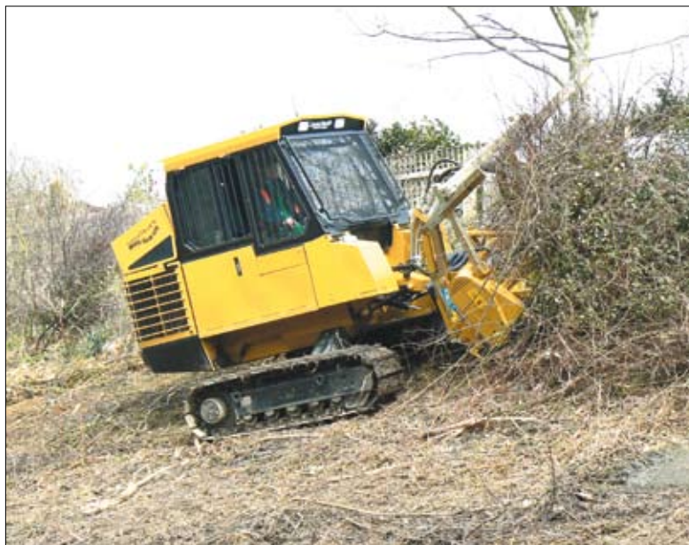
The Multi-Task 120 clearing the way through neglected embankments.
