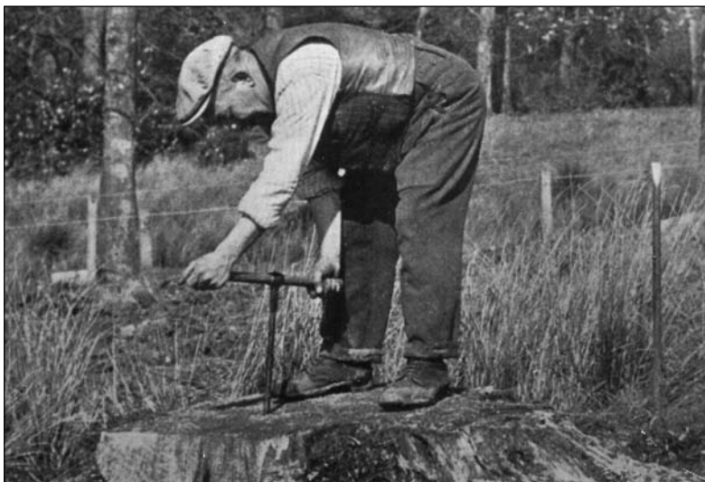
(Left) Boring a hole with a hand auger to set explosives. (Right) A line explosion – the quickest way to clear a ditch in pre-excavator days. (It probably still is!)
