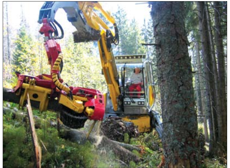
The Menzi Muck, which is normally supplied with the Woody 50 head.
