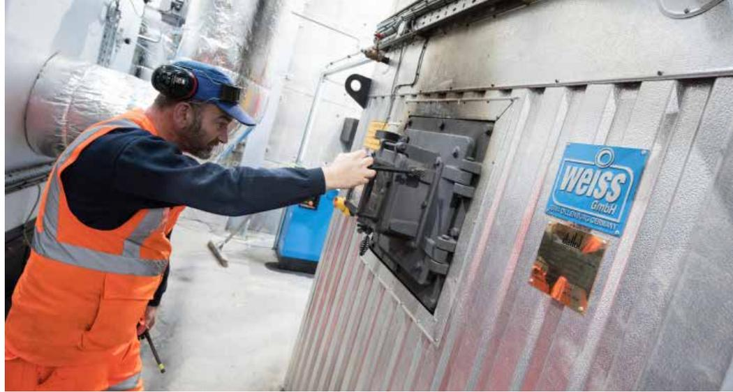
Above: The Weiss boiler supplies hot water to the kiln-drying operation.
